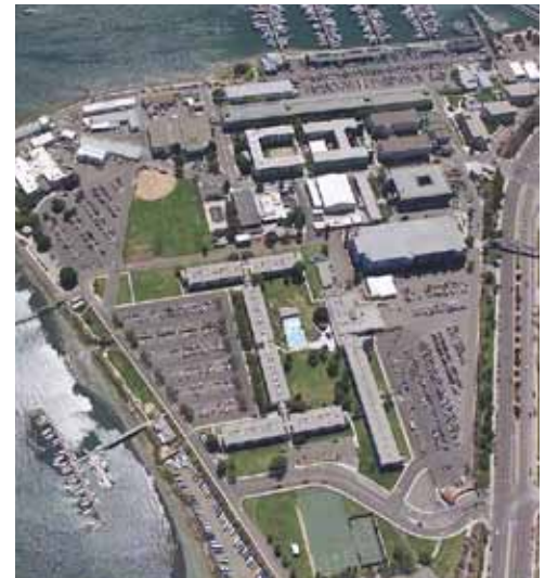
NMAWC COMPLEX, NAVAL BASE PT. LOMA
