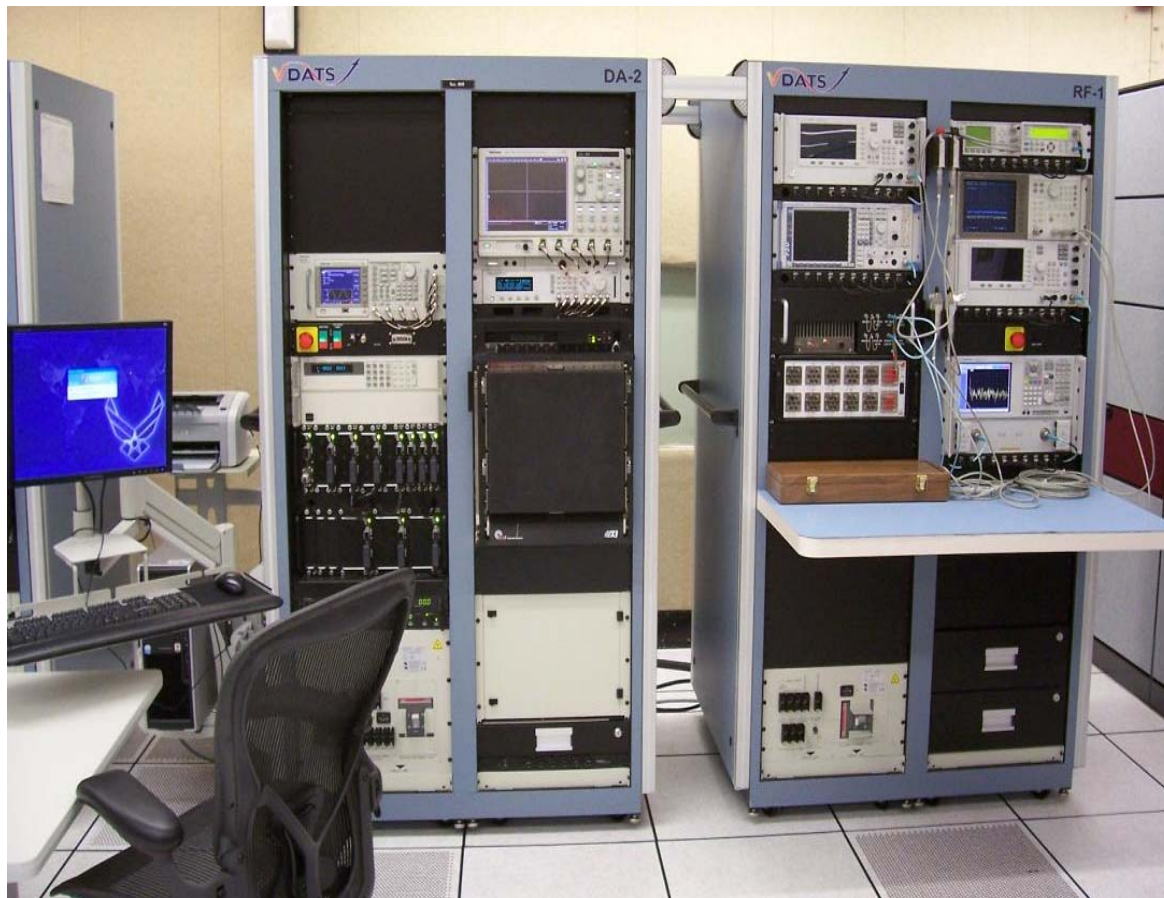
VDATS DA-2 with RF Auxiliary Unit
