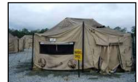
Improved Temporary Facilities Insulation
